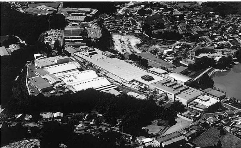
KITZ Nagasaka Plant, Japan
