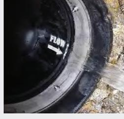
The CheckMate® Valve will crack open and flow with as little as 1" of head pressure.
