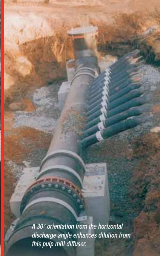
A 30° orientation from the horizontal discharge angle enhances dilution from this pulp mill diffuser.
