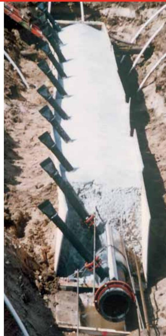
One hundred, twenty nine 4" Tideflex® valves with 16" square flanges were retrofitted over original 2" fixed-orifice ports on a reinforced concrete outfall in California.
