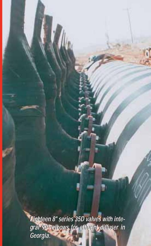
Eighteen 8" series 35D valves with integral 90° elbows for effluent diffuser in Georgia.
