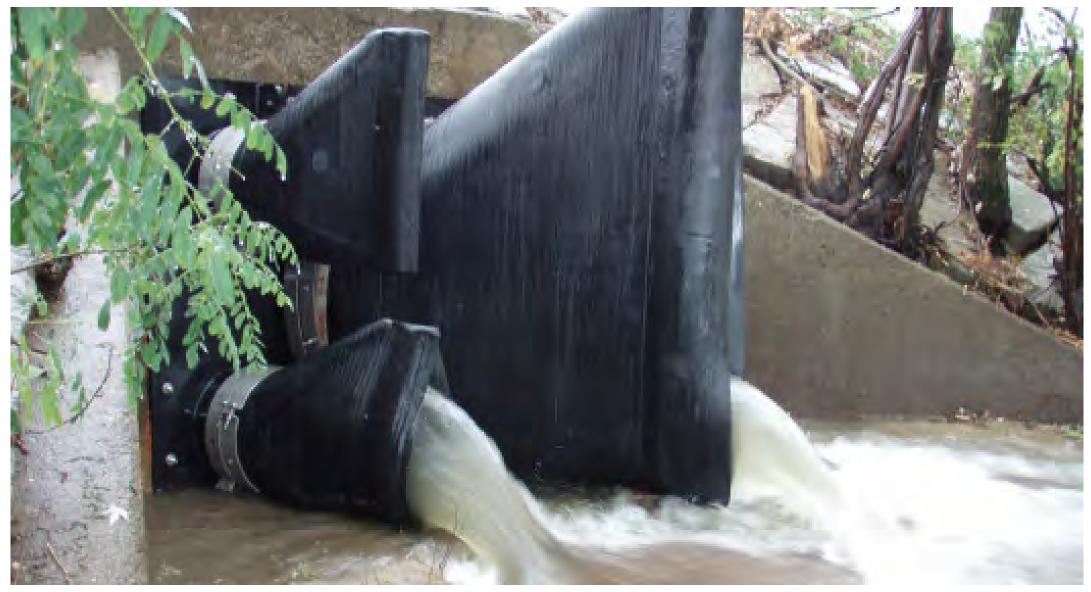
Red Valve products are used in combined sewer overflow (CSO), sanitary and SSO systems to protect unwanted backflow flowing into storm water catchments during times of rising rivers, high tide and heavy rainfall. When these systems overflow, excess wastewater containing untreated human and industrial waste, toxic material, and debris is discharged directly into streams, rivers, and lakes.
