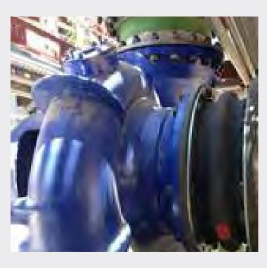
**Redflex®** Expansion Joints absorb vibration, compensate for pipe misalignment and movement. They help alleviate piping stress, compensate for movement, reduce noise and isolate vibration. Red Valve offers flanged and slip-on connections, single or multiple arches and a range of elastomers to meet process conditions, including Teflon®-lined joints for severely corrosive applications.
