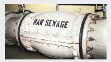
The Type A Control Valve is highly effective handling concentrated sewage and abrasive grit, which often moves at a considerable velocity as it enters the treatment process.
