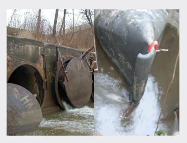
Problem: Traditional flap gate valves get stuck open, allowing millions of gallons of water to go back into systems or treatment plants for re-treating.
