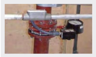
**Red Valve Pressure Sensors** are used to protect pumps from running dry or over pressuring the line by providing accurate, dependable pressure movement. With full 360° pressure reading, Red Valve sensors are the only sensors that will stay operational on difficult process fluids such as sewage, sludge, and scum.
