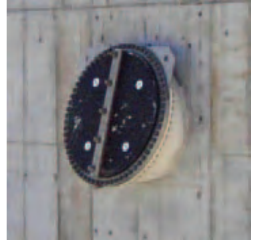
This 84" Waterflex was installed in the inlet tower of an 1100 acre reservoir.
