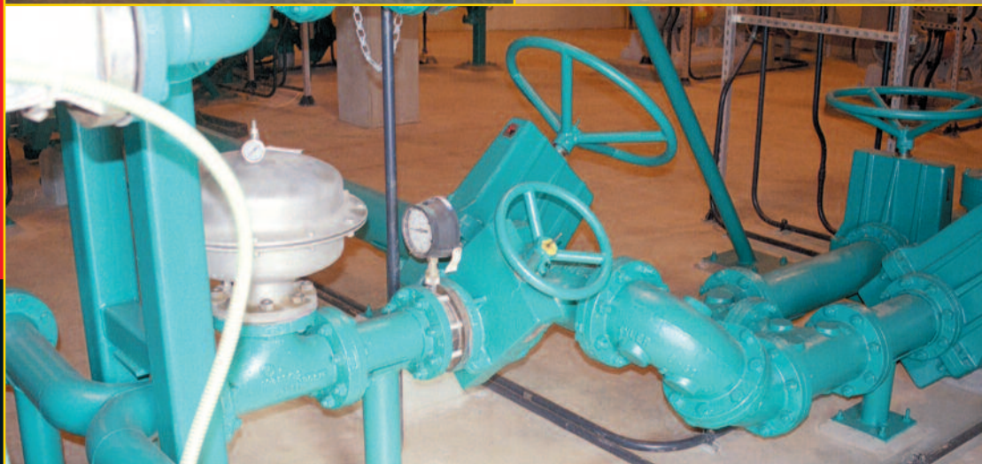
Electrically operated Series 5400E controls digester sludge accurately and requires no maintenance.
