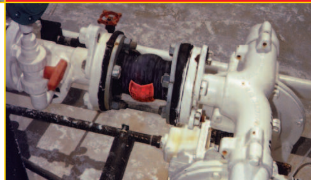
Right: Filled arch J-1 Redflex Expansion Joint on lime pumping system.
