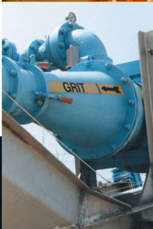
Near right: Series 40 pressure sensors can withstand the rigors of grit removal.
