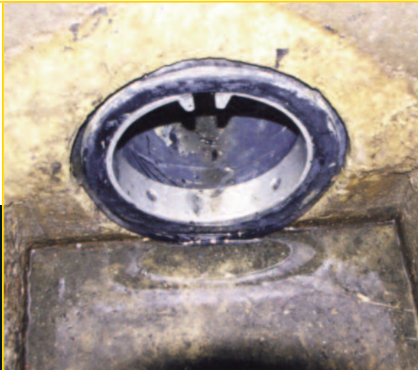
Engineered rubber check valves have memory: forward hydraulic pressure opens the valve, and reverse pressure seals the valve and prevents backflow.
