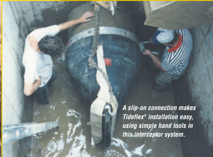
Engineered rubber check valves have memory: forward hydraulic pressure opens the valve, and reverse pressure seals the valve and prevents backflow.
