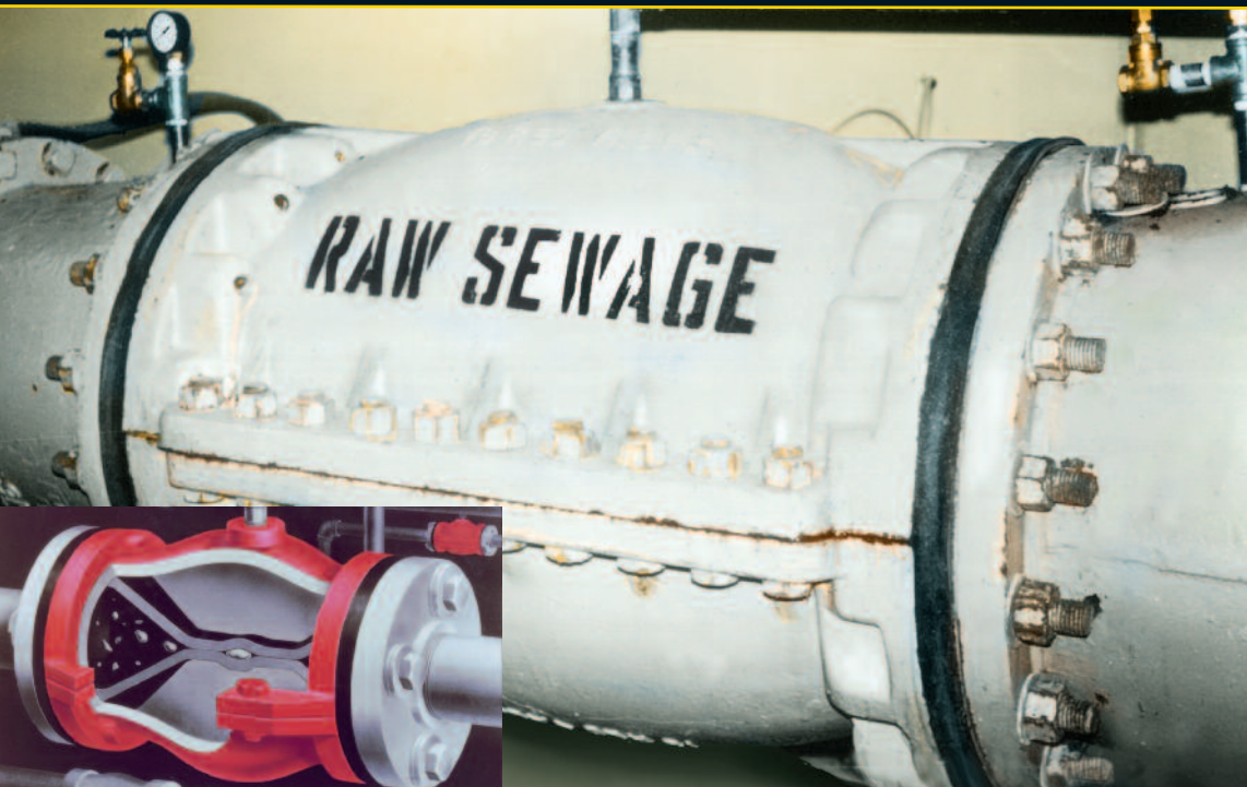
Left: Type A pinch valves are the only automated valves that need no actuator and close drop-tight on solids.
