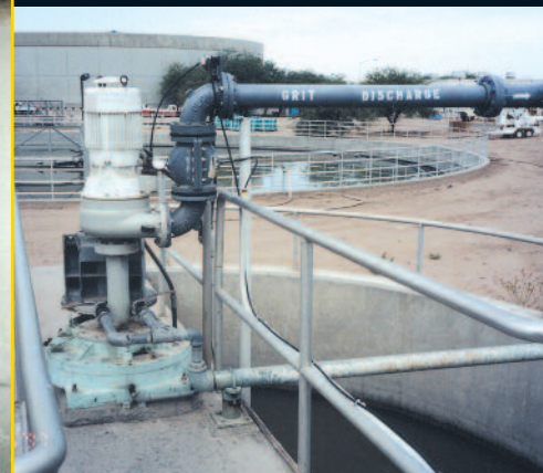
Left: Type A pinch valves are the only automated valves that need no actuator and close drop-tight on solids.
