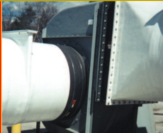
Above: Large diameter square and round ducting joints on an air handling system.
