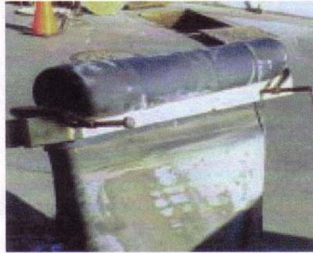
Place a 2 x 4 on either side of the bill, and use C-clamps to hold tight while adhesive sets.
