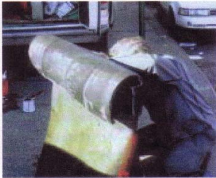
Slide extension onto bill, and fasten with stainless steel screws* spaced one inch apart.
