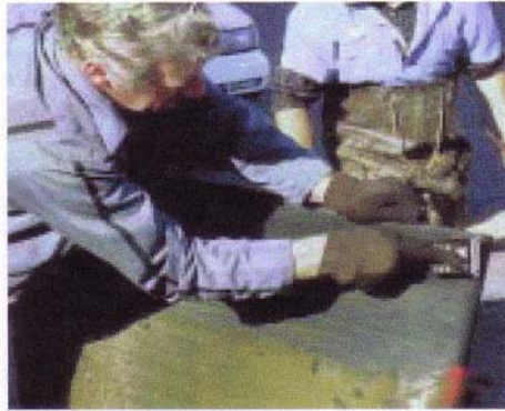
Remove hard deposits with metal scraper, wire brush, or angle grinder.
