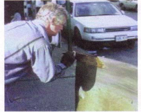
Prepare surface with thinner or toluene. Apply adhesive* around entire circumference of bill.
