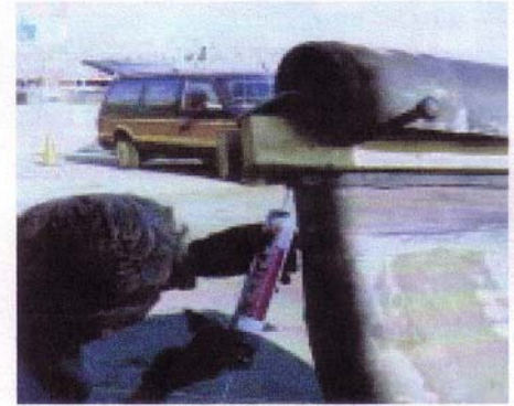
Silicone caulk can be applied along the edge of the bill for extra protection.
